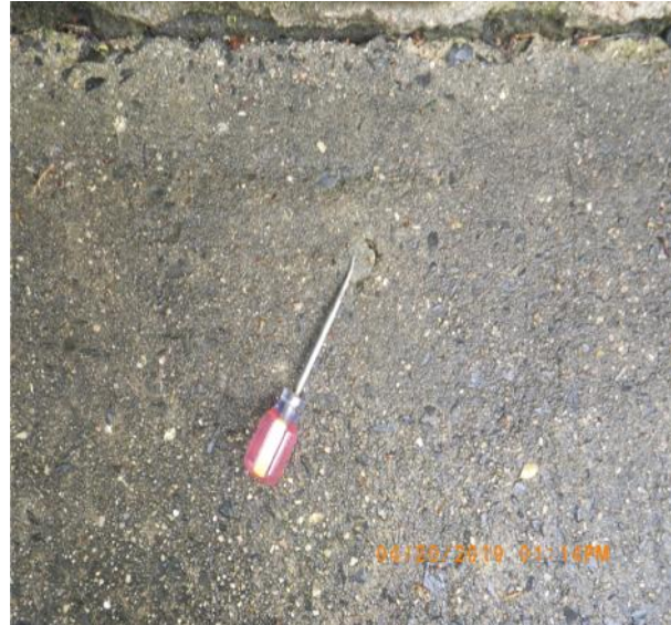
abc235 (44).JPG Termite treatment-Drill marks from previous termite treatment by another company.
