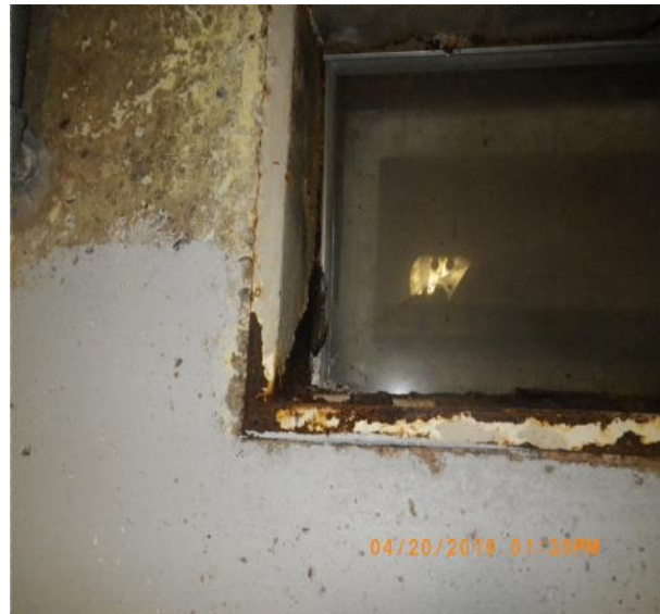
abc235 (54).JPG Replace rear basement window (excessive damage to window frame and cracked window glass).
