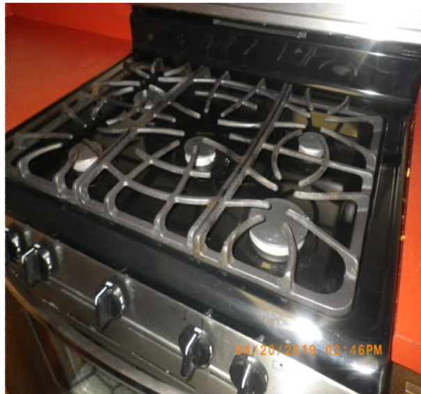
abc235 (73).JPG Range-Repair non-operating gas range burners (burner would not ignite, safety hazard).
