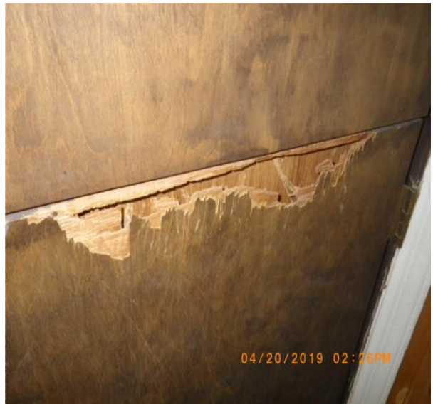
abc235 (68).JPG Replace damaged door in the laundry room.
