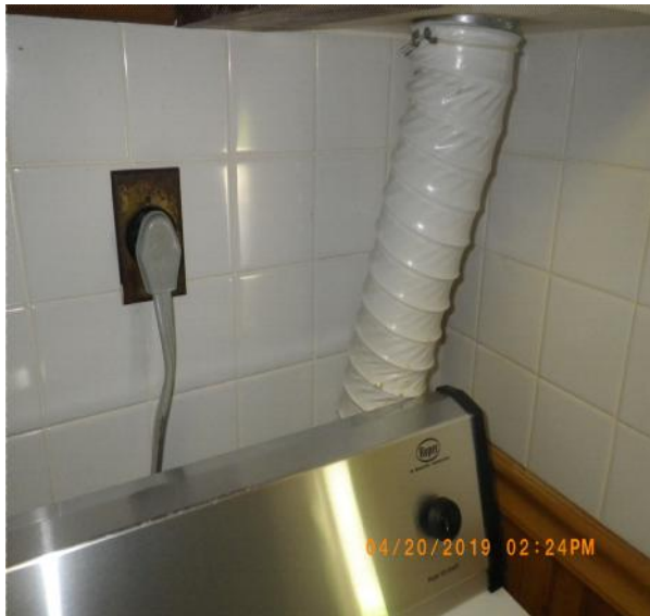
abc235 (67).JPG Replace gas dryer vinyl vent hose with metal vent pipe (fire hazard).
