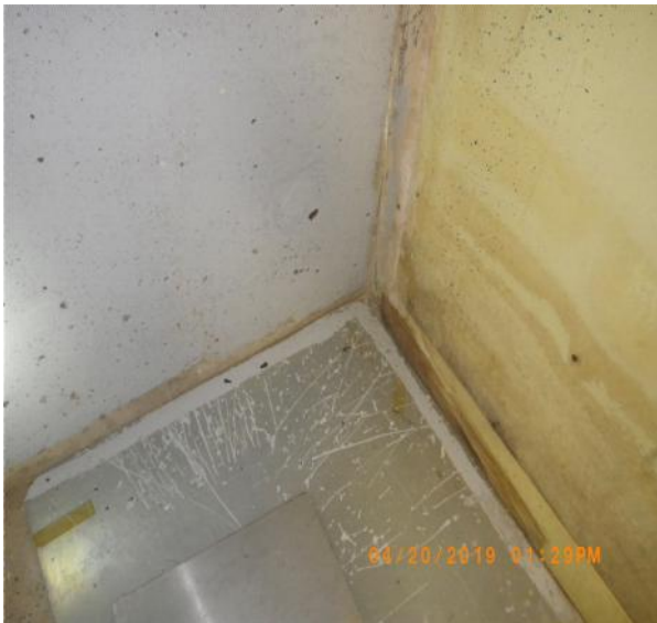
abc235 (53).JPG Contractor specializing in basement waterproofing should examine signs of exterior water penetration into the basement noted on rear basement wall and repair as needed.
